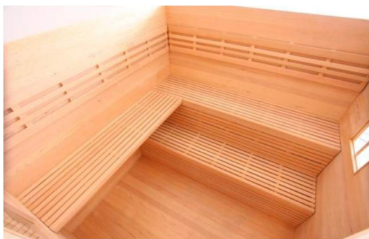
Figure A-6: Installing the 2 layers of bench
